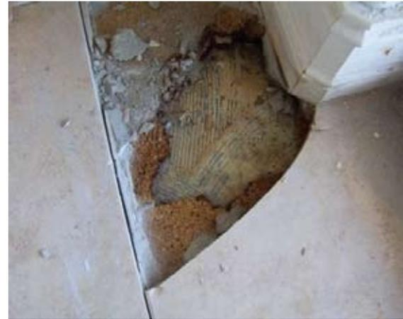
**Above: The stained grout in this installation was removed following water seepage from a nearby window.**
